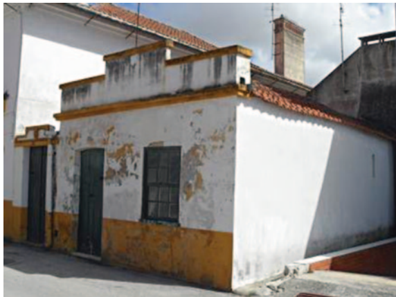
Fig. 15 Old building with reinforced concrete elements (credit A. Tavares)
