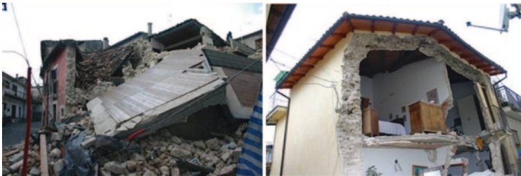
Fig. 7 Damage caused by past interventions, Abruzzo 2009
