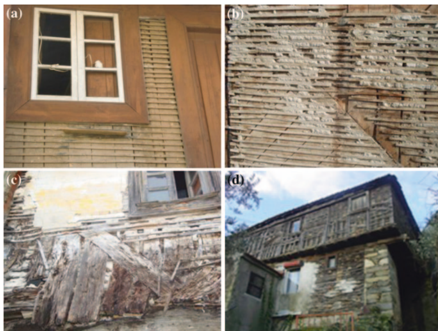
Fig. 2 Timber structural system typologies of tabique walls. a Typology 1. b Typology 2. c Typology 3. d Typology 4
