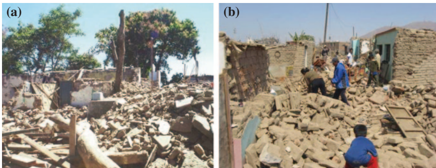
Fig. 6 Destruction of adobe houses due to earthquakes. a EI Salvad 2004 [4]. b Pisco, Peru 2007
