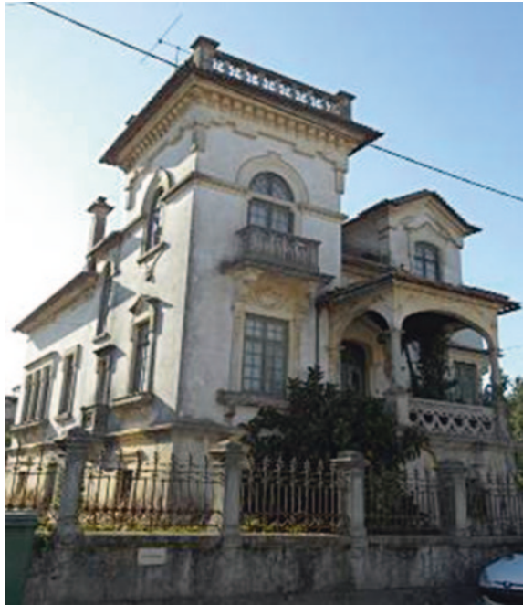
Fig. 9 Adobe construction in Portugal (credit A. Tavares)
