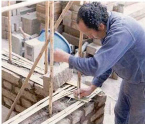
Fig. 27 Internal cane mesh reinforcement [77]
