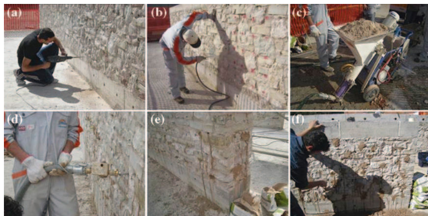
Fig. 8 Grout injection on stone masonry walls [4]: a drilling holes for the injection; b cleaning the drilled holes by blowing compressed air; c injection pump machine; d injection of a wall; e grout mixture leaking from a “control” hole; f sealing of the hole with mortar
