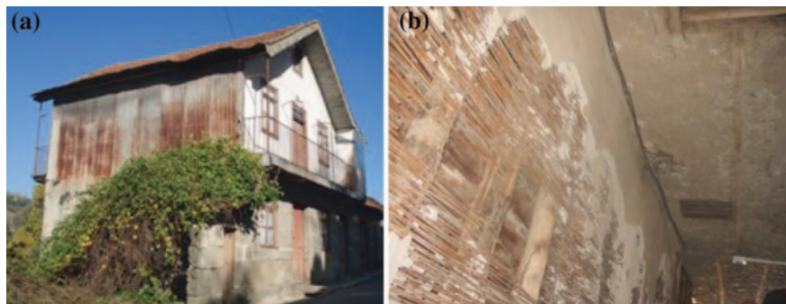
Fig. 1 Examples of tabique dwellings. a Portuguese ( exterior view ). b Turkish ( interior view )
