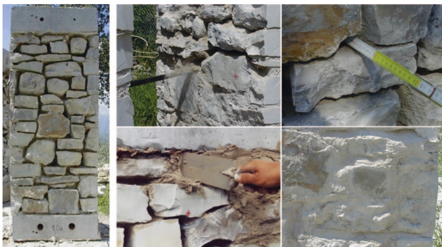
Fig. 9 Deep re-pointing procedure [7]
